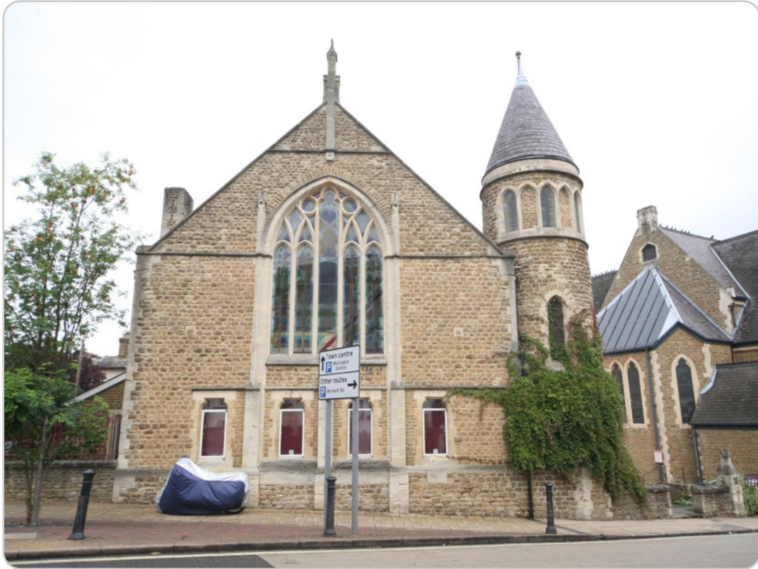
Wesley Hall (east end) Barrack Road, Aldershot
