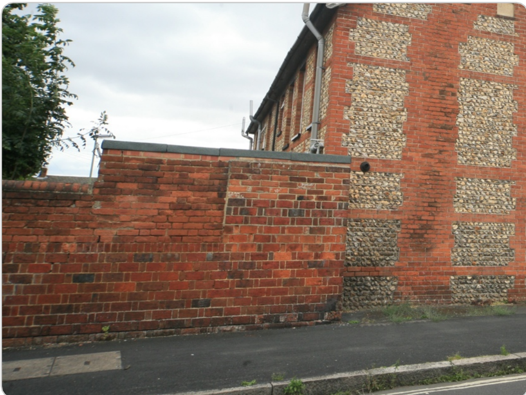
Boundary wall to Nos.33-39 (W side) Brighton Road, Aldershot
