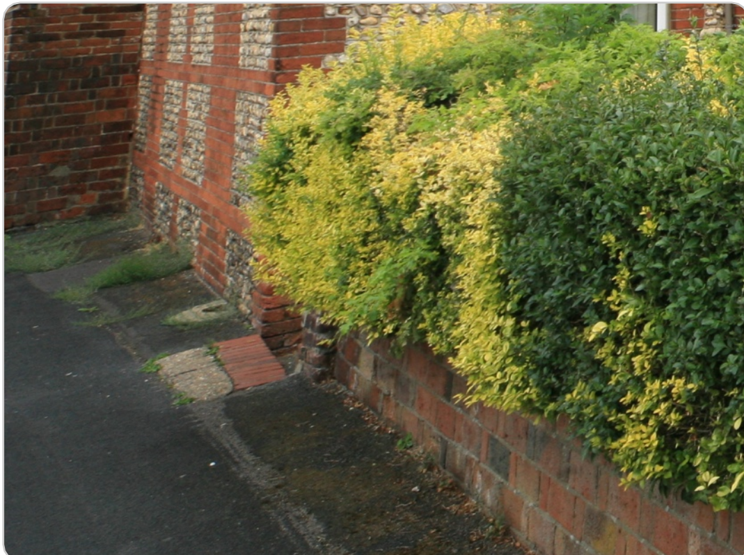
Boundary wall to Nos.33-39 (W side)
