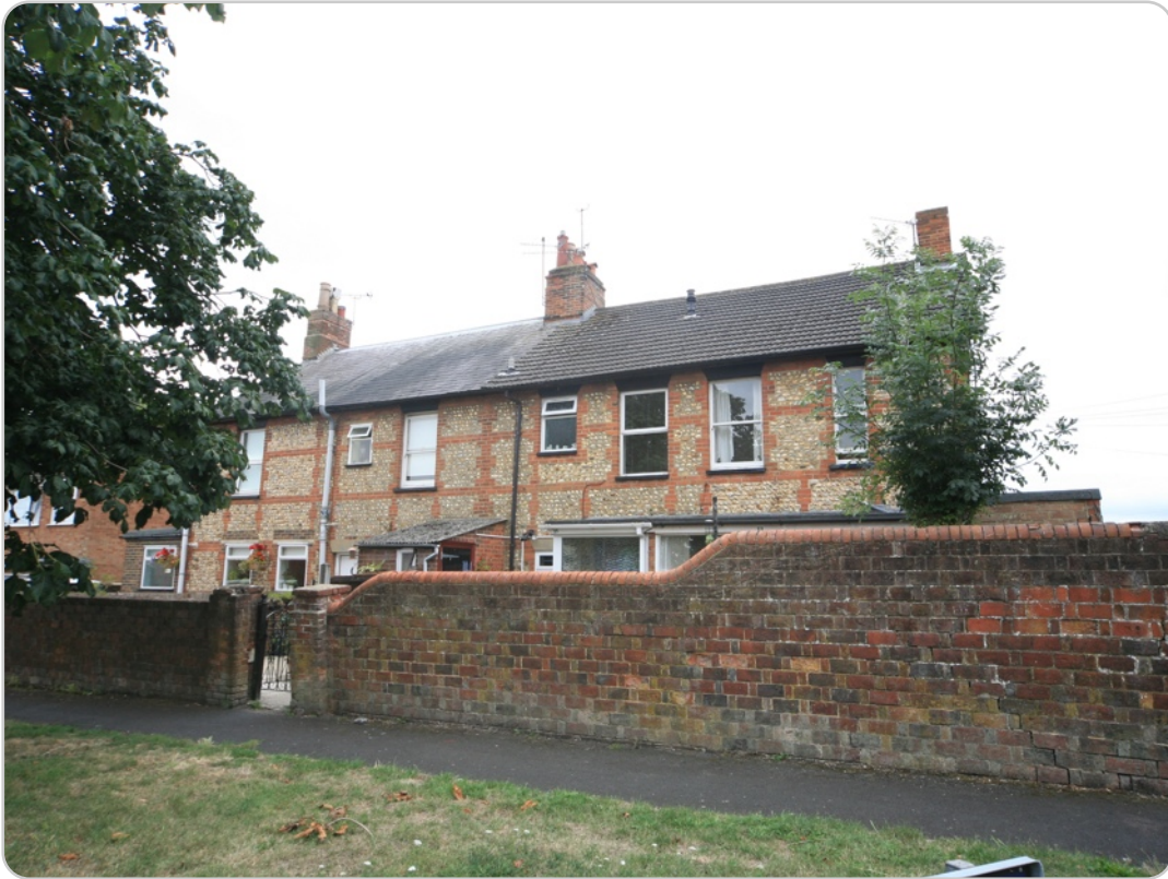
Boundary wall to Nos.33-39 (N side) Brighton Road, Aldershot
