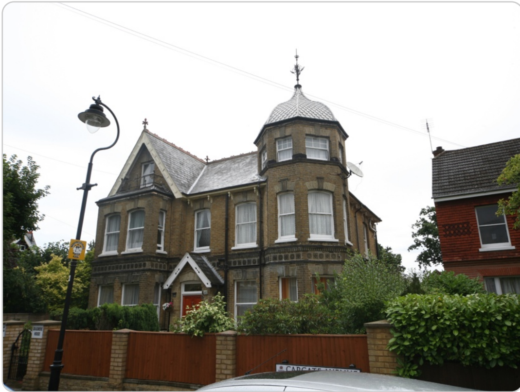
Grasmere House (SW corner)
