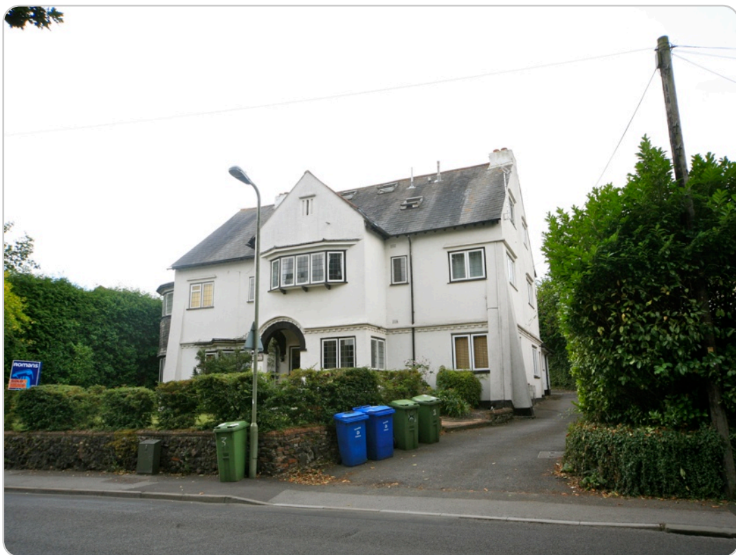
The Glebe House (NE elevation)
