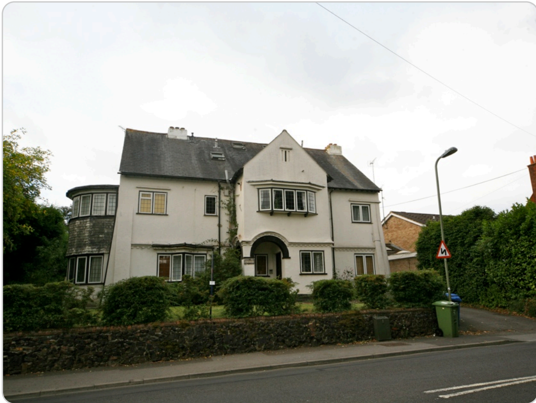
The Glebe House (NE elevation)
