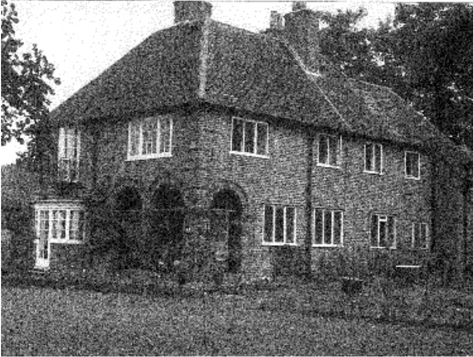
Albury Barn, Church Lane West, Aldershot (HRO)
