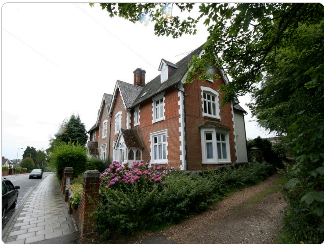
91 Tall Chimneys & No.93 (NW corner) Cranmore Lane, Aldershot
