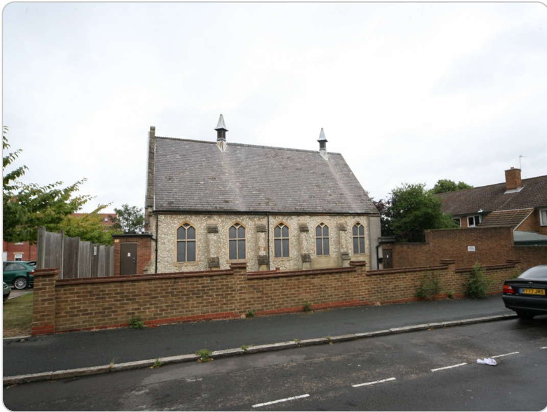
Masonic Hall (S elevation) Edward Street, Aldershot
