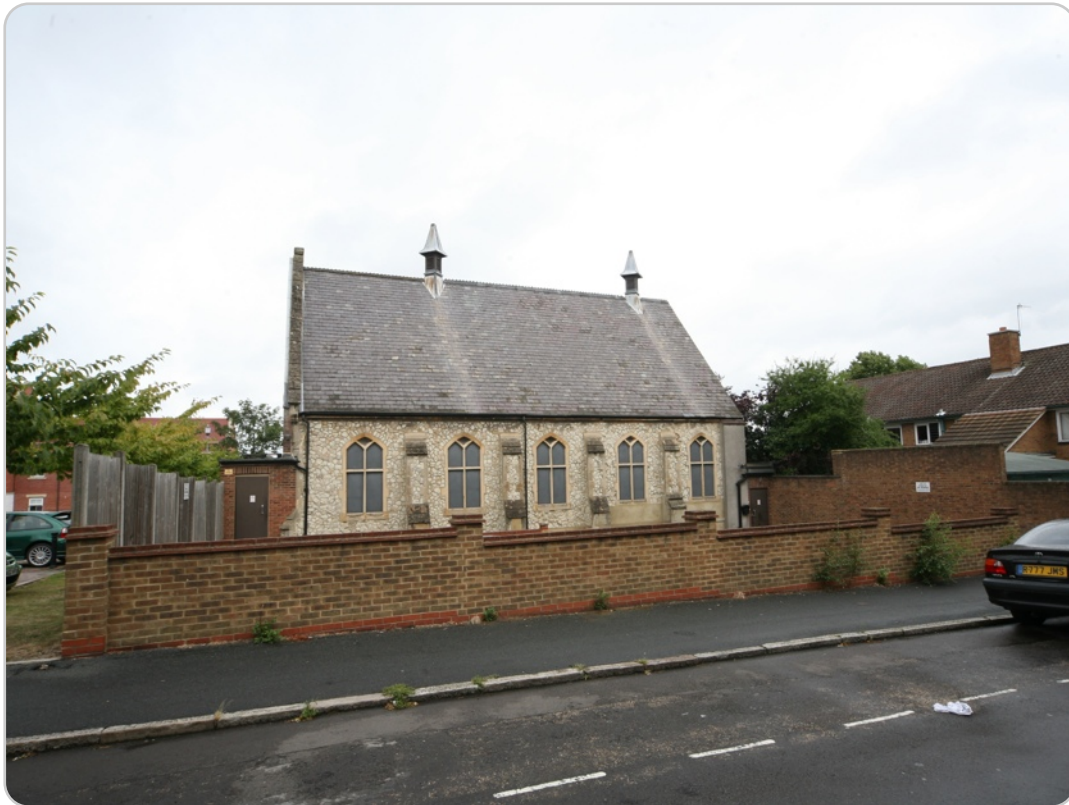
Masonic Hall (S elevation) Edward Street, Aldershot
