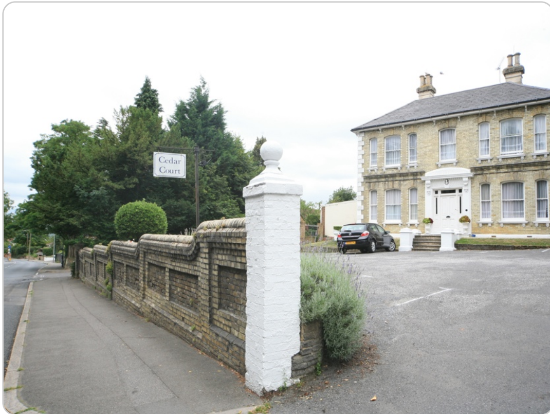
Boundary wall to Cedar Court (E elevation)
