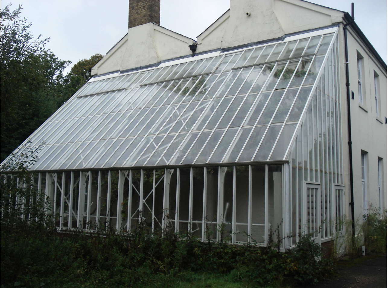
Vine Cottage, 3 Farnborough Road, Aldershot - south elevation and viney
