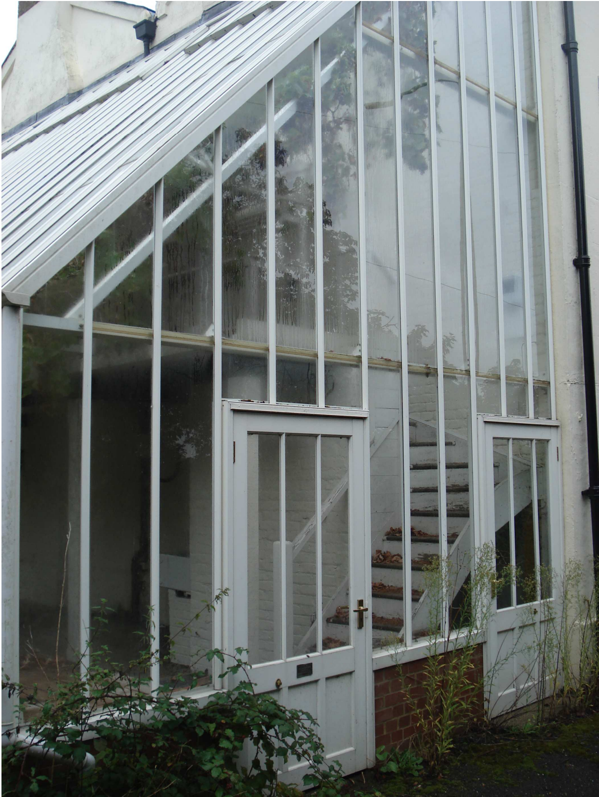
Vine Cottage, 3 Farnborough Road, Aldershot - south elevation (detail of vinery)
