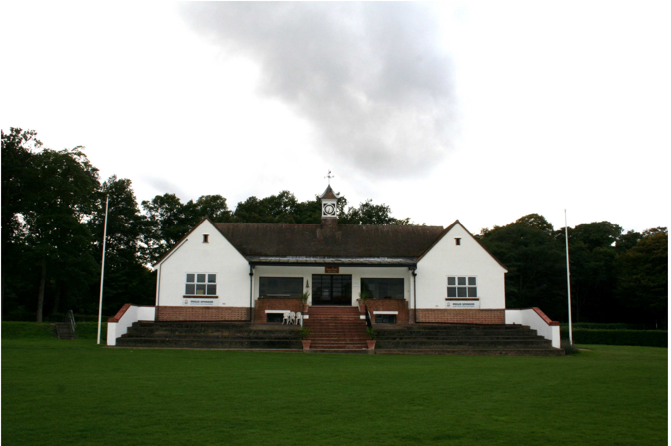
Army Cricket Pavilion, Fleet Road, Aldershot – South elevation
