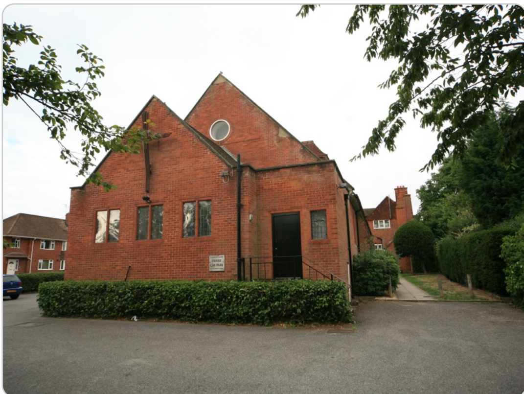
St Augustines Church (E end) Holly Road, Aldershot
