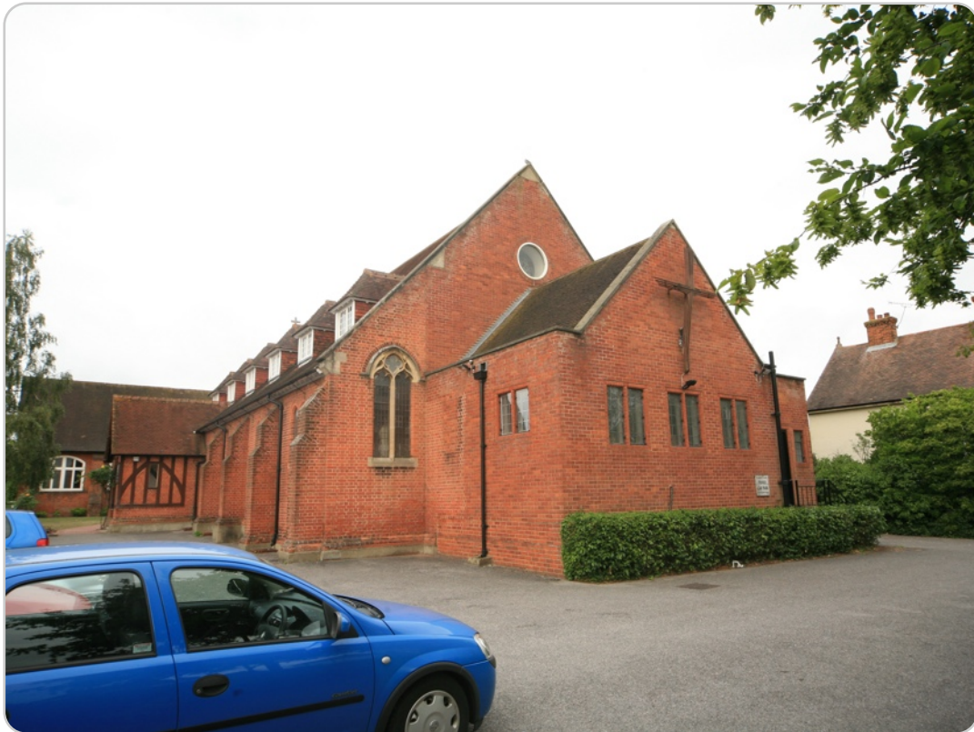
St Augustines Church (SE corner) Holly Road, Aldershot
