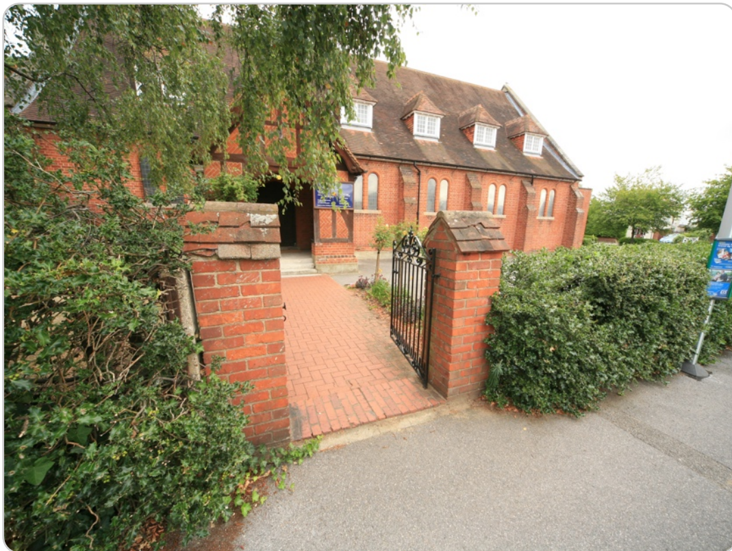
St Augustines Church (Boundary Wall) Holly Road, Aldershot
