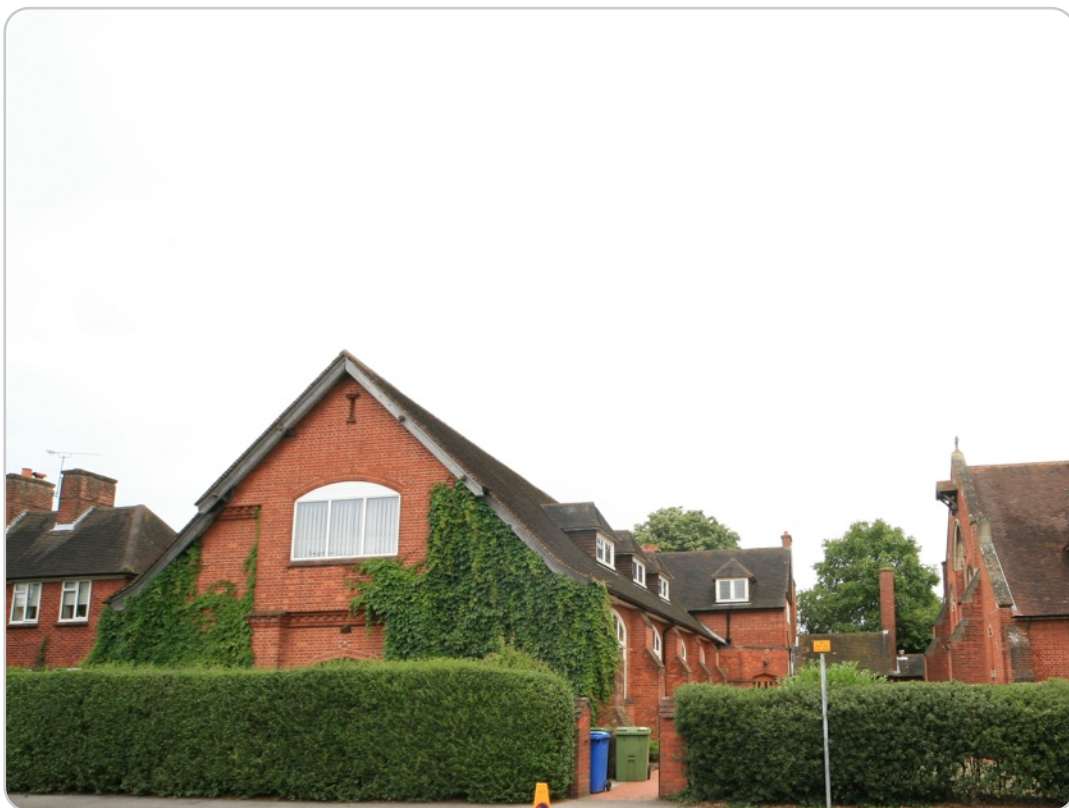
St Augustines Church (S elevation) Holly Road, Aldershot
