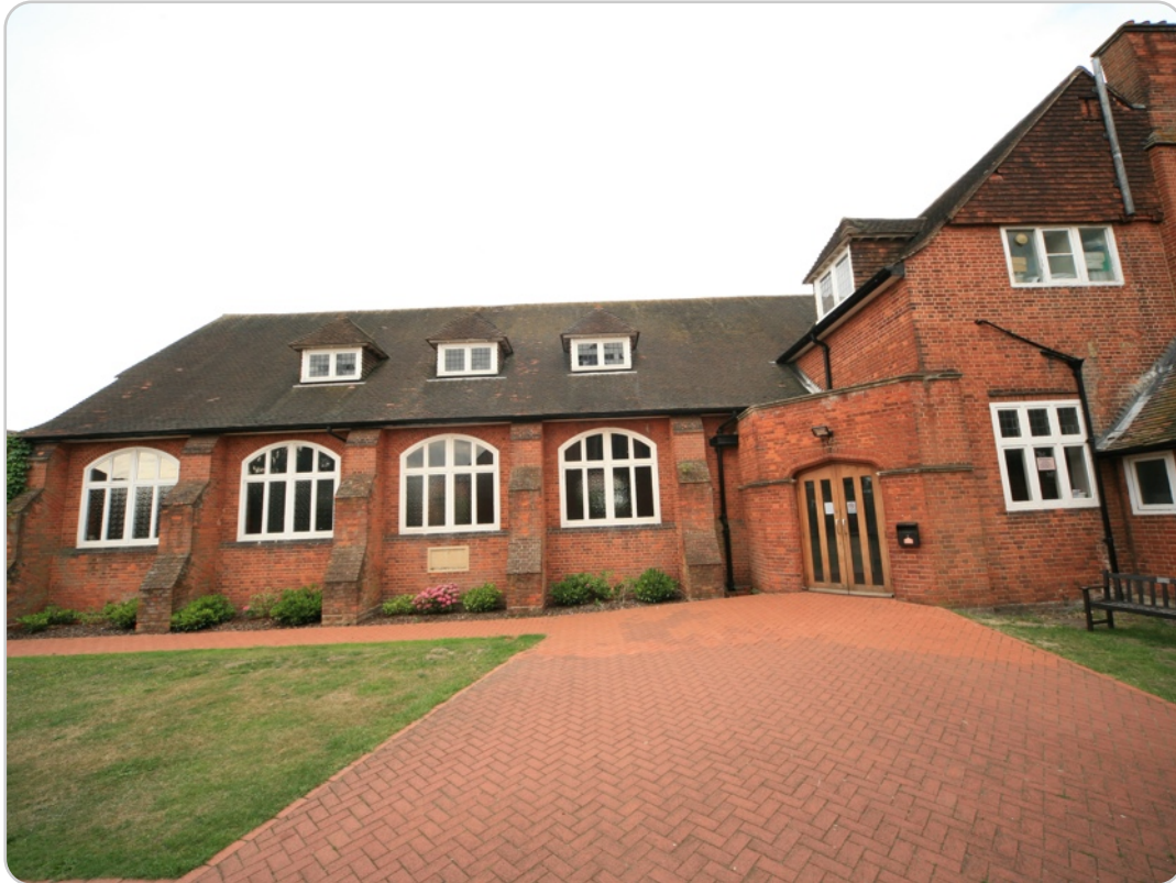
St Augustines Church Hall (E elevation) Holly Road, Aldershot
