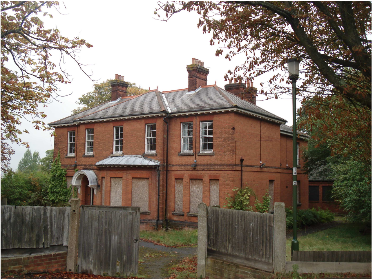
Cambridge House, Hospital Road (North side), Aldershot – South elevation
