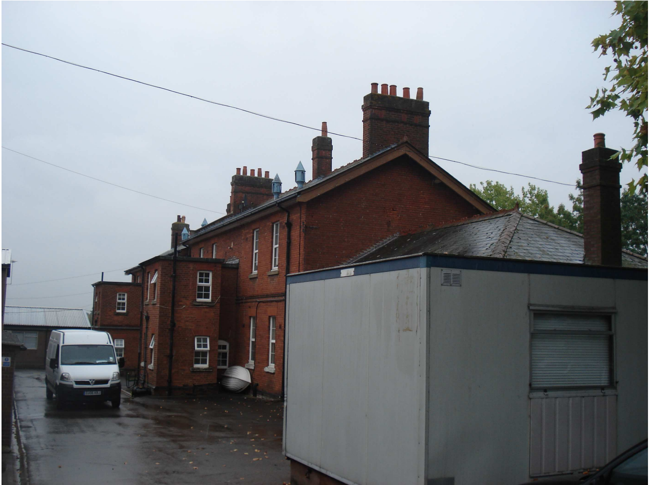
Military Police Barracks Block, Headquarters, Steeles Road, Aldershot
