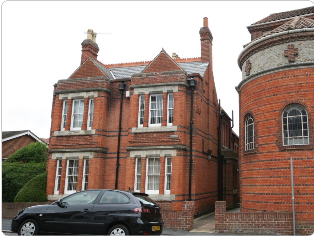
St Joseph's Rectory (S elevation) Queen's Road, Aldershot
