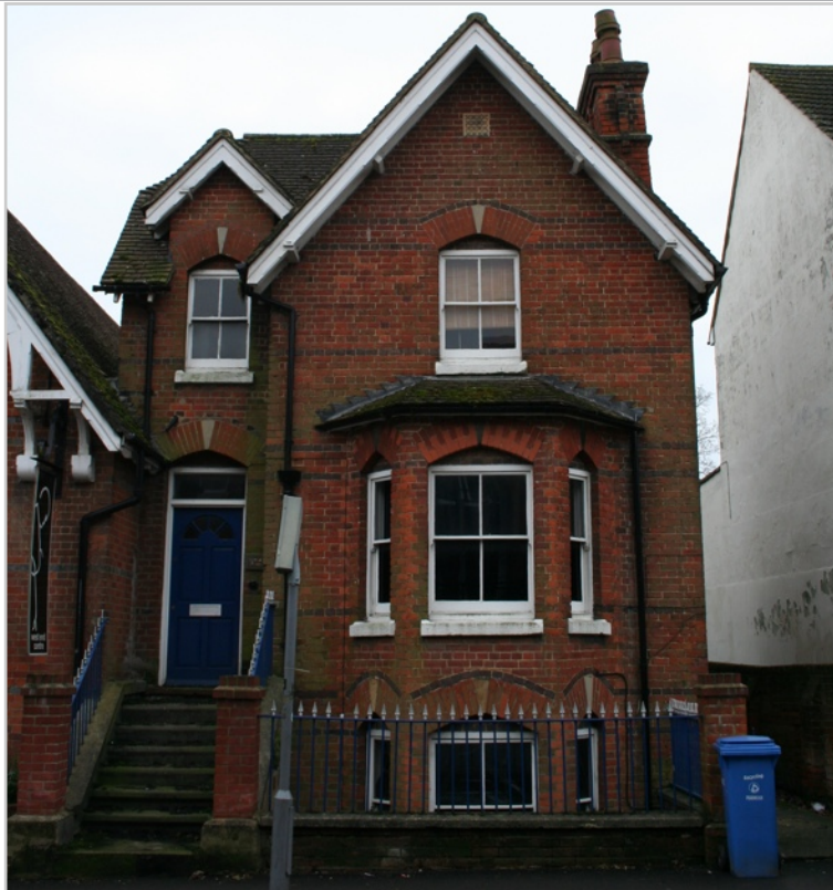
The West End Centre (N elevation W end) Queen's Road, Aldershot
