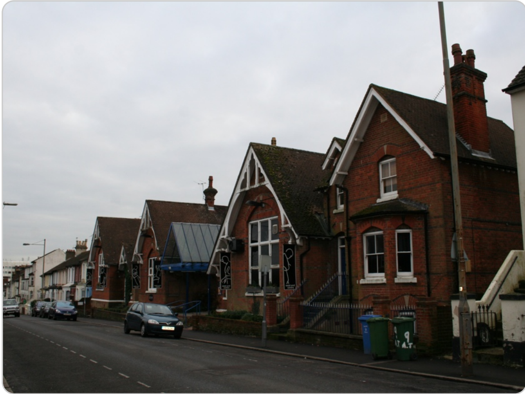
The West End Centre (N elevation)
