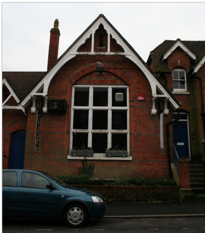
The West End Centre (N elevation W end) Queen's Road, Aldershot
