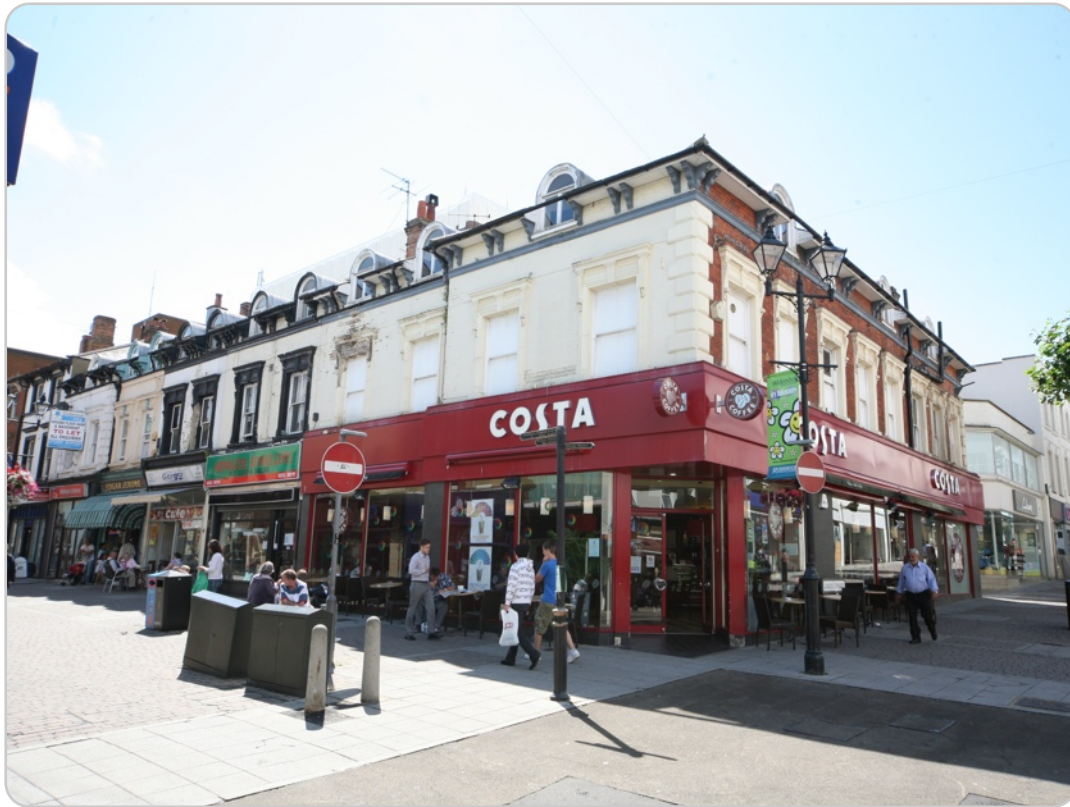
Nos. 49-51 Union Street, Nos.3-11 Wellington Street (N corner)
