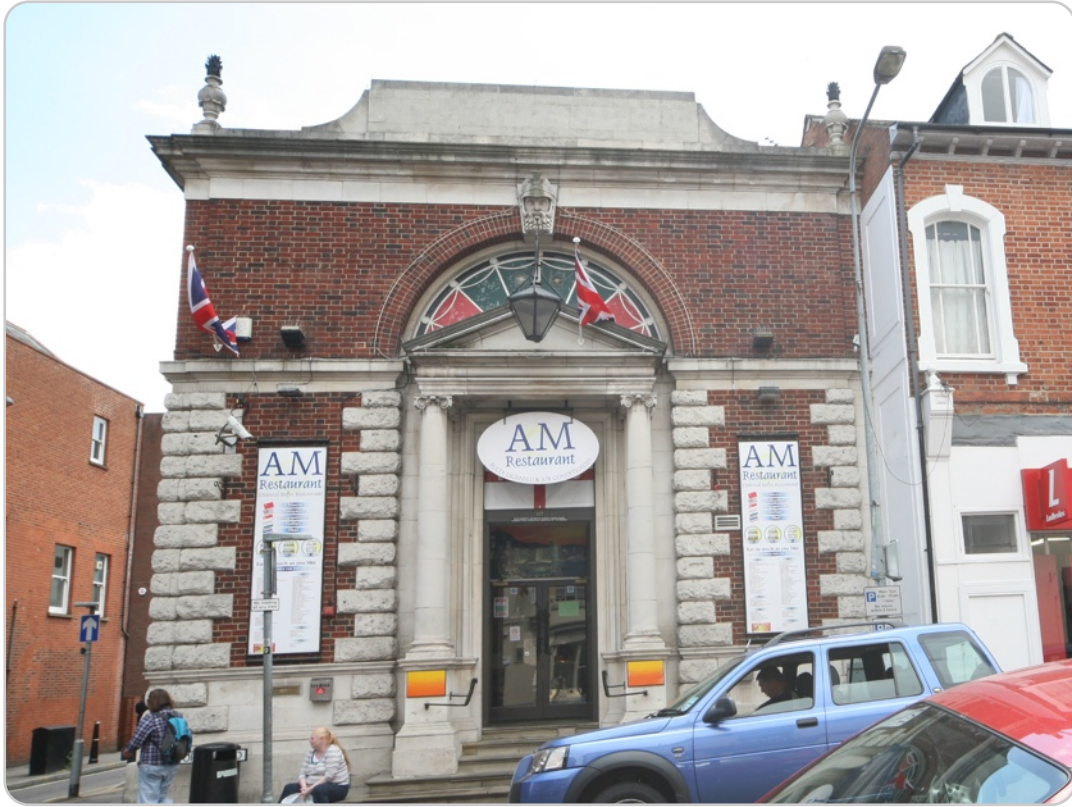
No.117 Victoria Road (N elevation)
