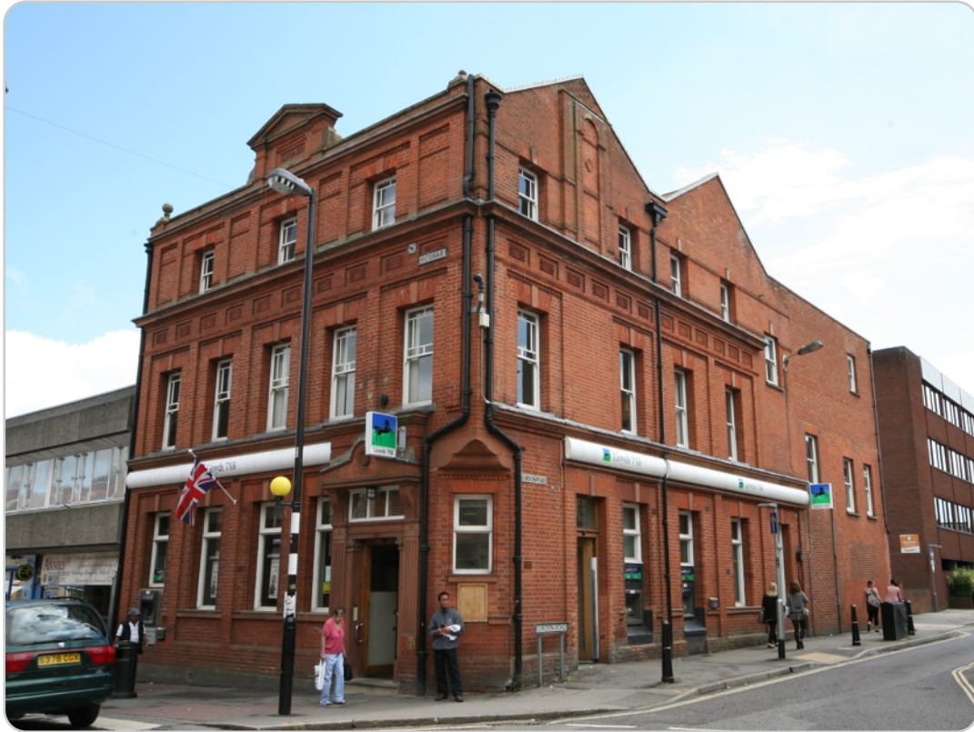
Lloyds Bank (NW corner)
