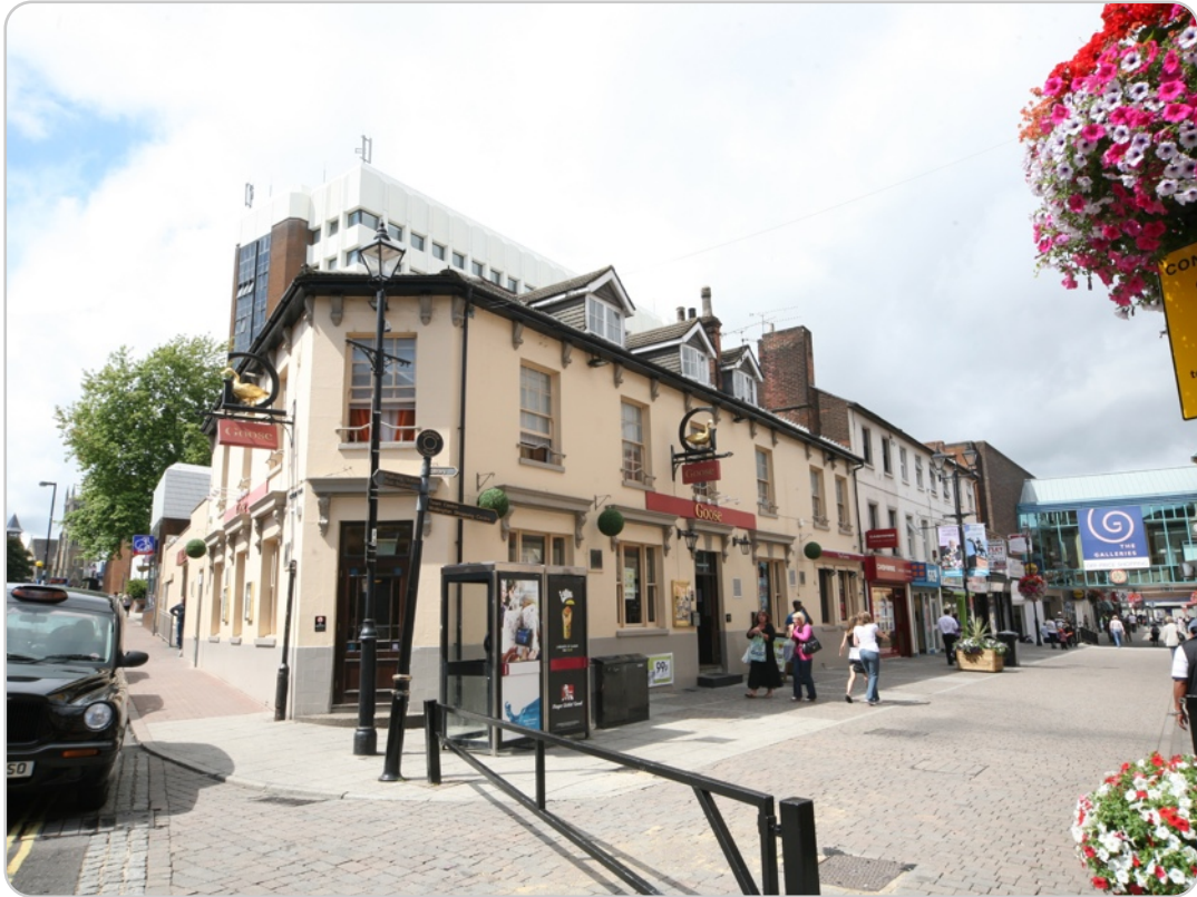
The Goose at Aldershot (SE corner)
