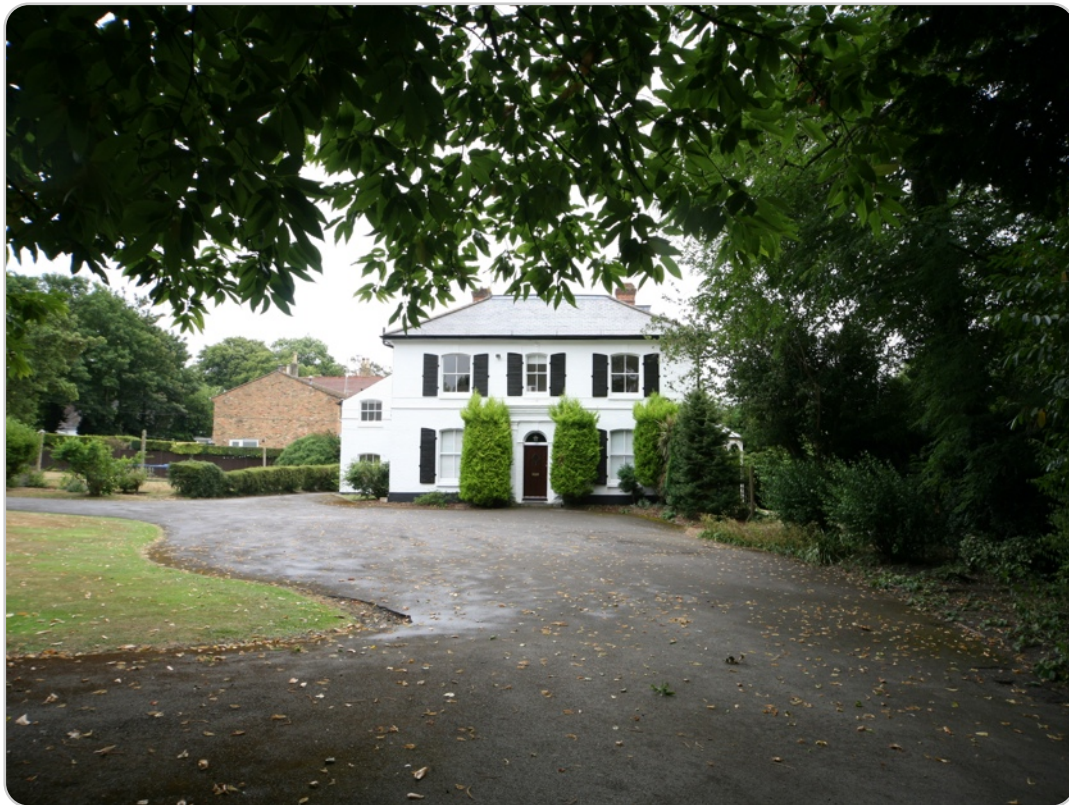
Normanton House (W elevation)
