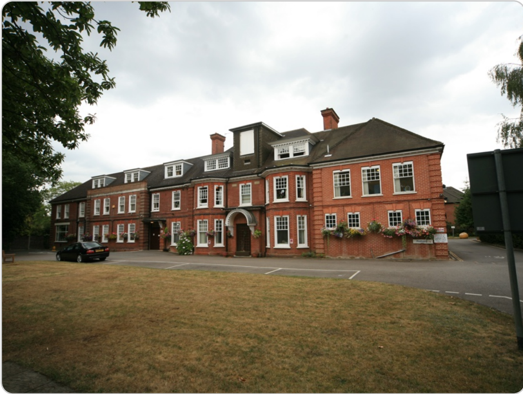
Devereux House (front elevation)
