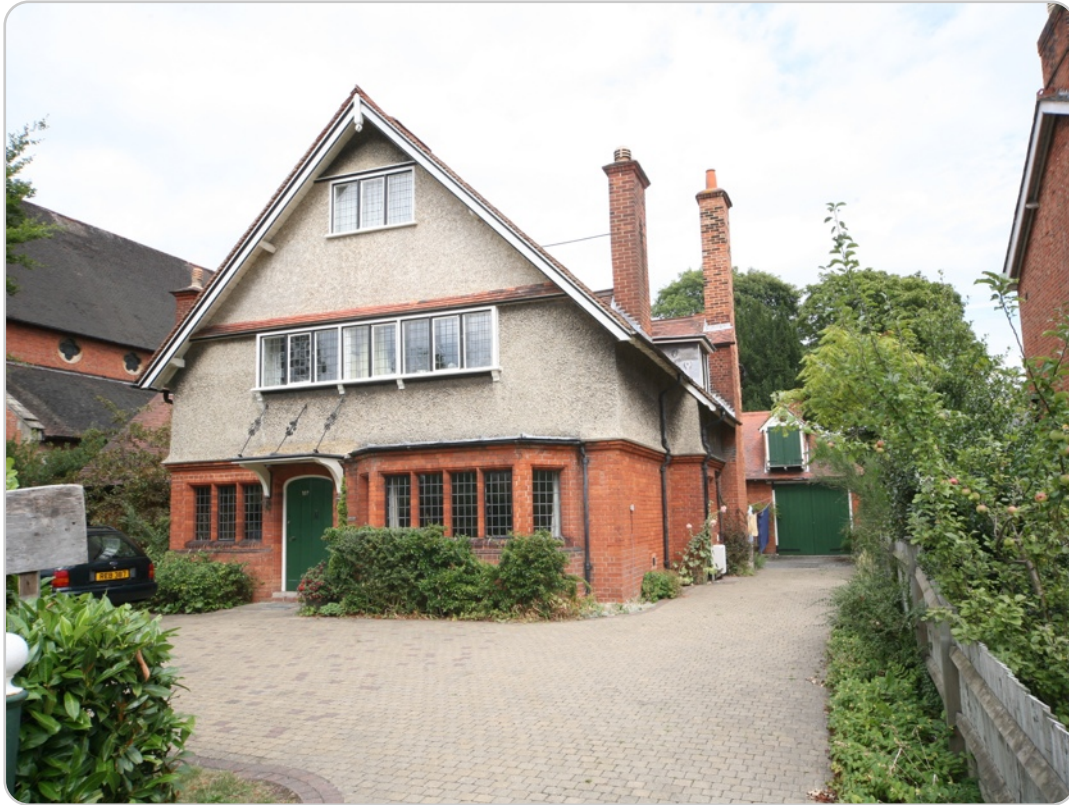
No. 107 (W elevation) Alexandra Road, Farnborough
