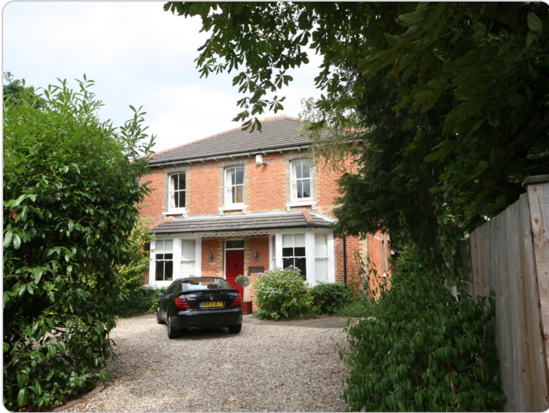
No. 63 Albany House (W elevation)
