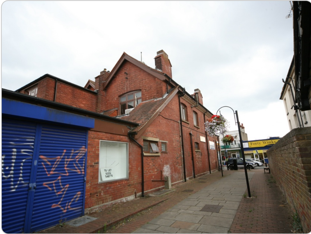
Former YMCA (N elevation)
