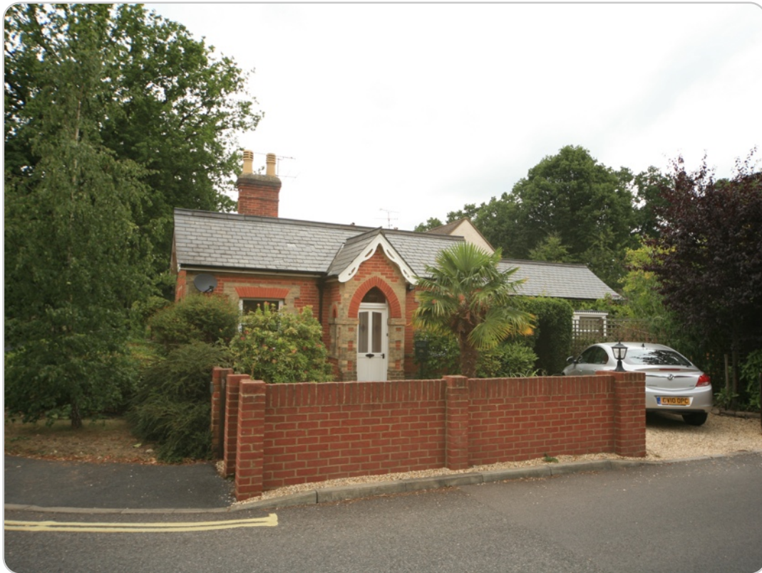
No.59 The Lodge (S elevation) Canterbury Road, Farnborough
