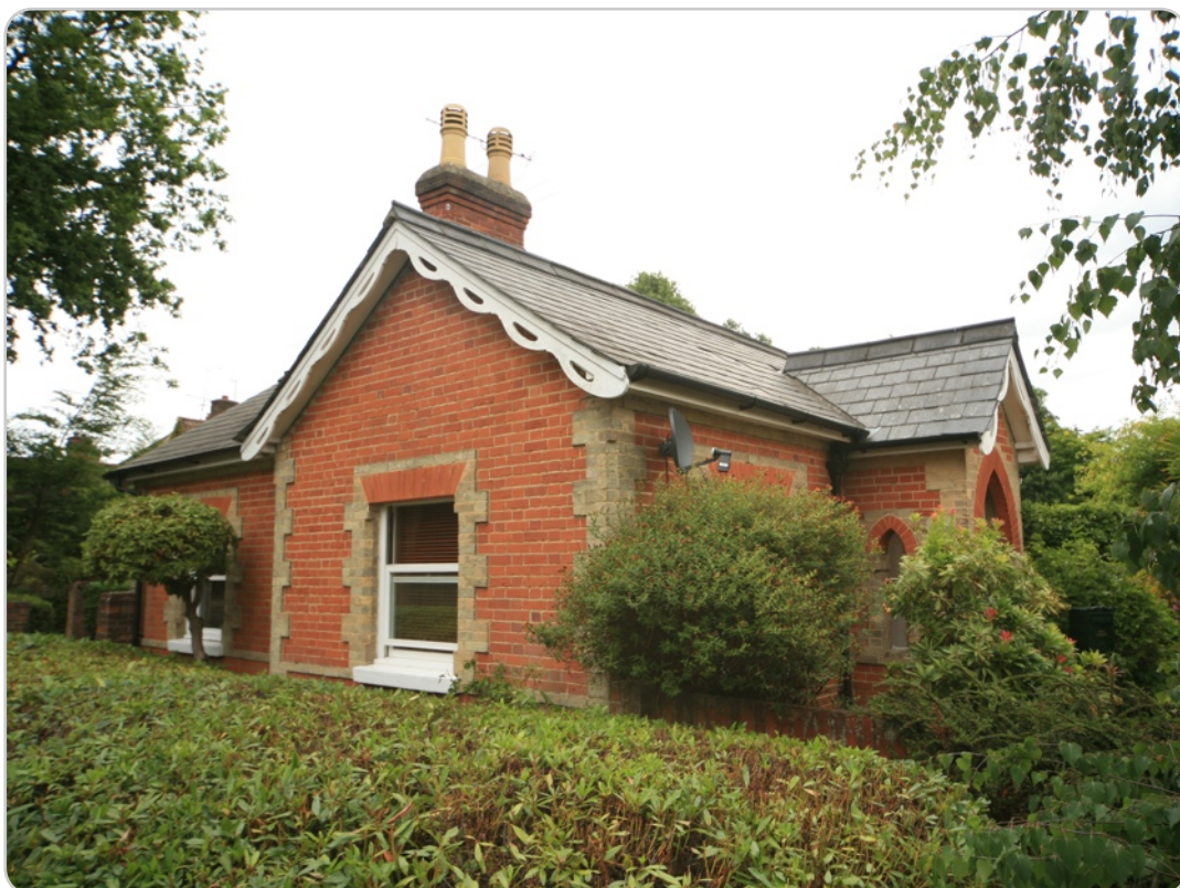
No.59 The Lodge (W elevation) Canterbury Road, Farnborough
