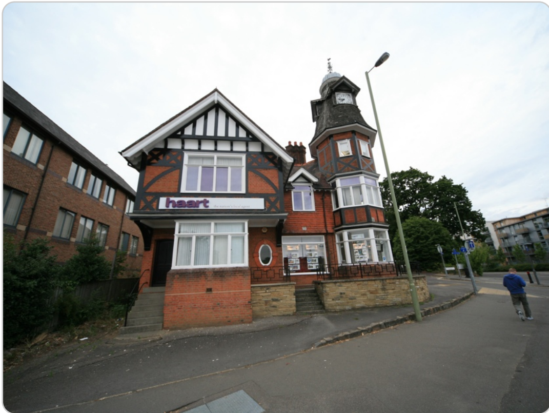
The Clockhouse (S elevation) Clockhouse Roundabout, Farnborough
