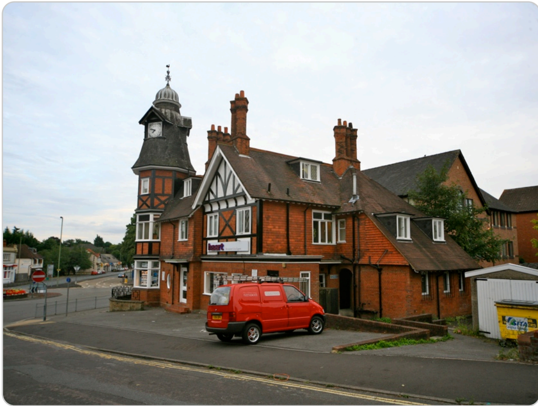
The Clockhouse (NE corner)
