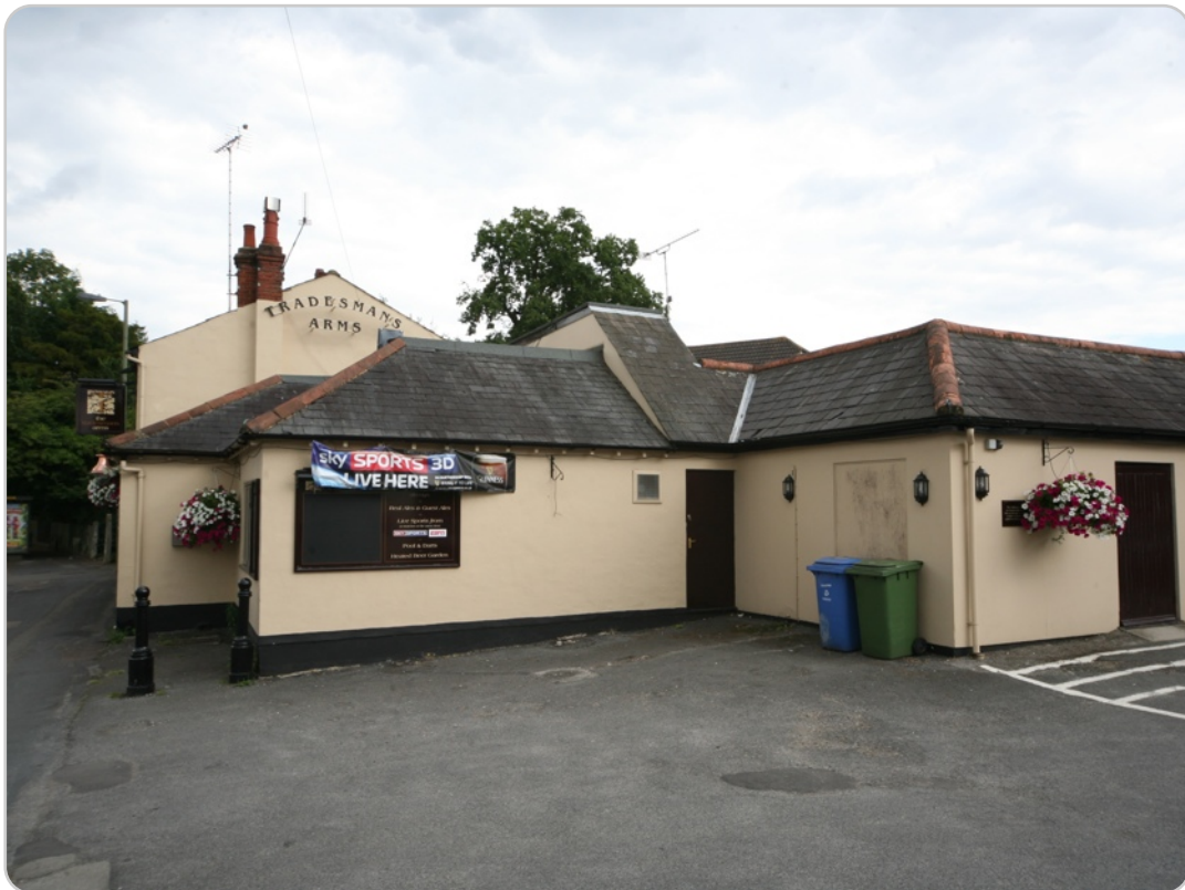
The Tradesmans Arms (W elevation) Cove Road, Farnborough
