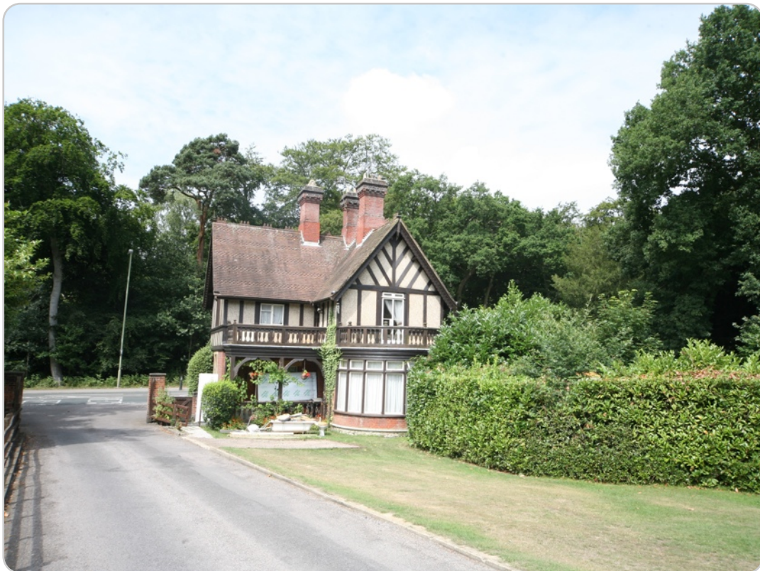
South Lodge (E elevation) Farnborough Road, Farnborough
