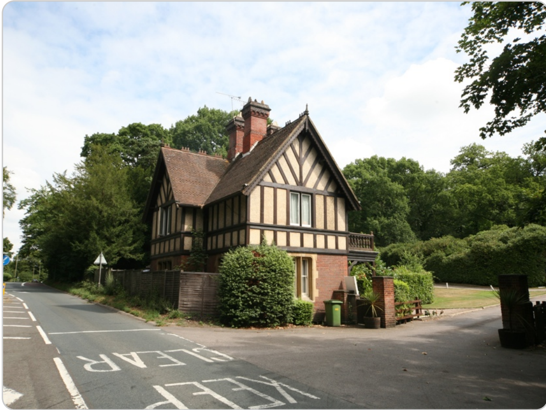
South Lodge (S elevation) Farnborough Road, Farnborough
