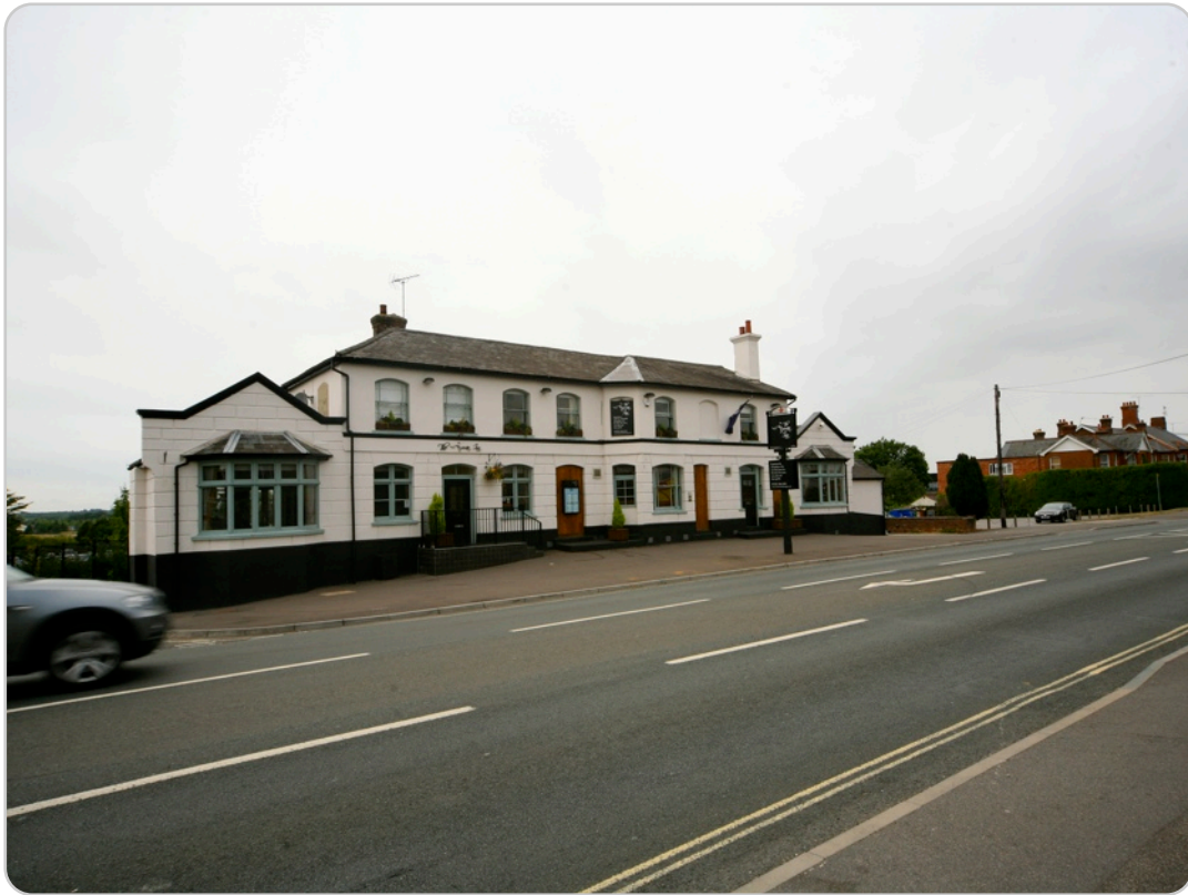
The Swan Inn (E elevation) 91 Farnborough Road, Farnborough
