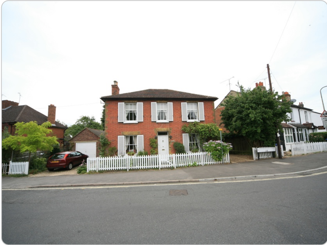
Elm Tree House (NW elevation) 9 Farnborough Street, Farnborough
