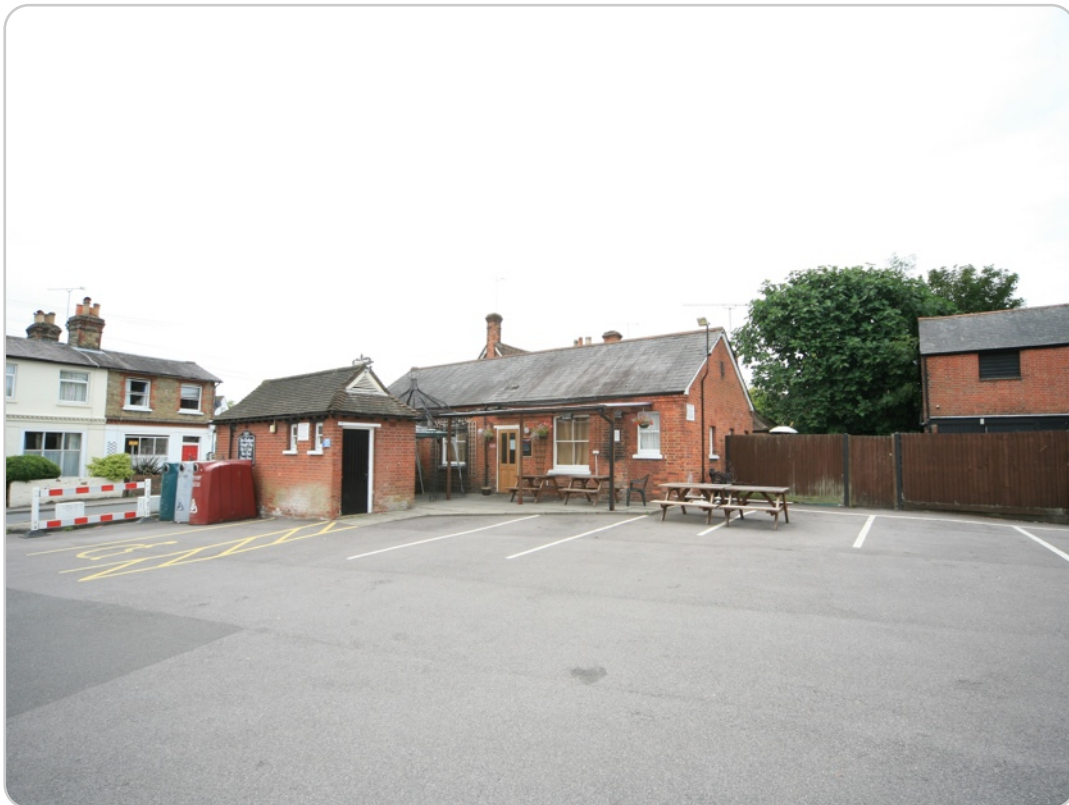
Imperial Arms PH (NE elevation) 12 Farnborough Street, Farnborough
