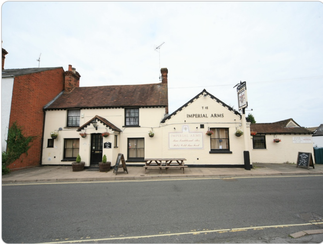
Imperial Arms PH (SE elevation) 12 Farnborough Street, Farnborough
