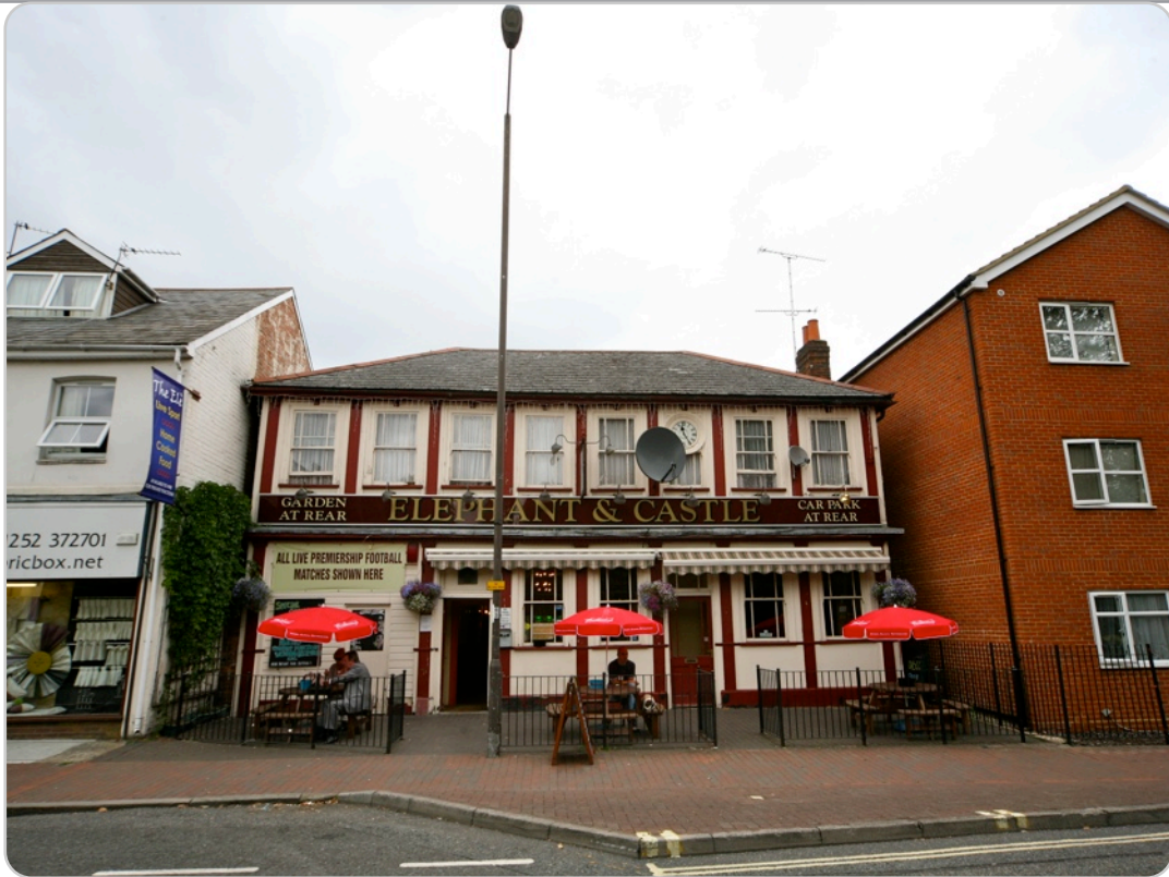
The Castle Inn (S elevation) 107 Lynchford Road, Farnborough
