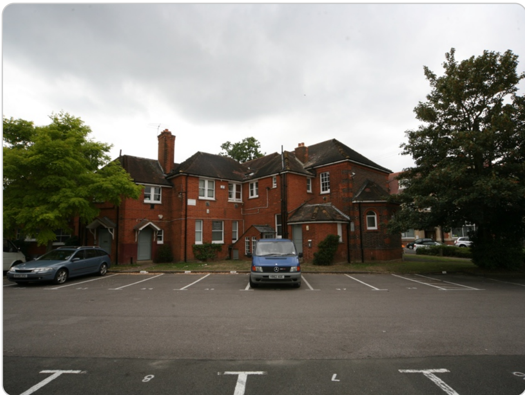
Old School Studios (E elevation) 40 Lynchford Road, Farnborough
