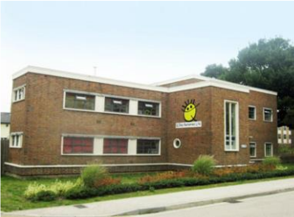
Building R170 (former Laundry) now Children's Nursery
