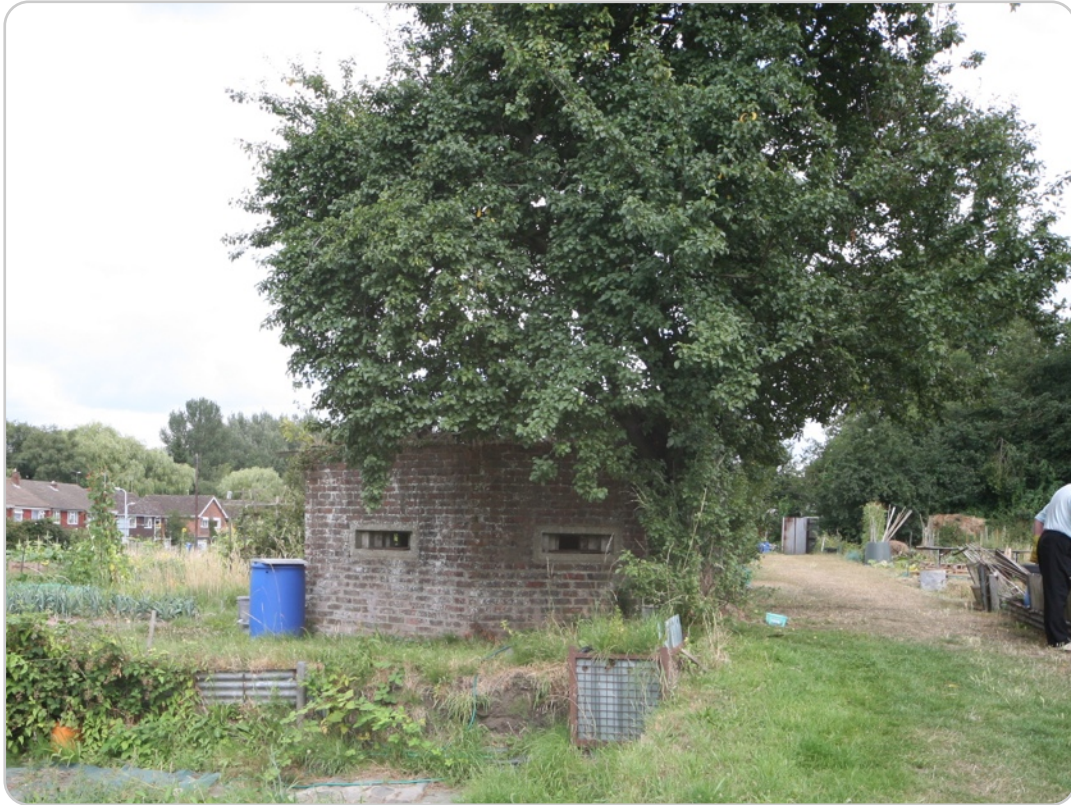
Pillbox Prospect Road, Farnborough
