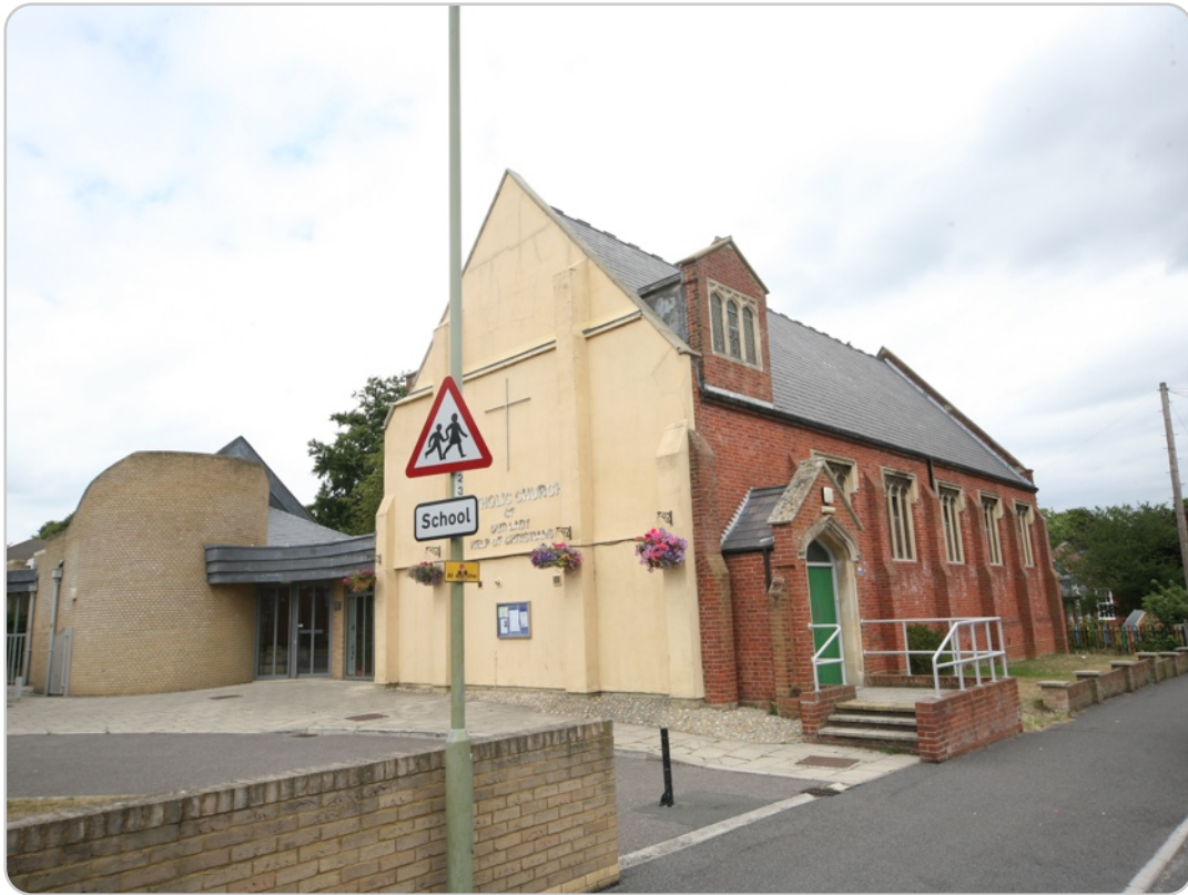
Church of Our Lady (SW corner) Queens Road, Farnborough
