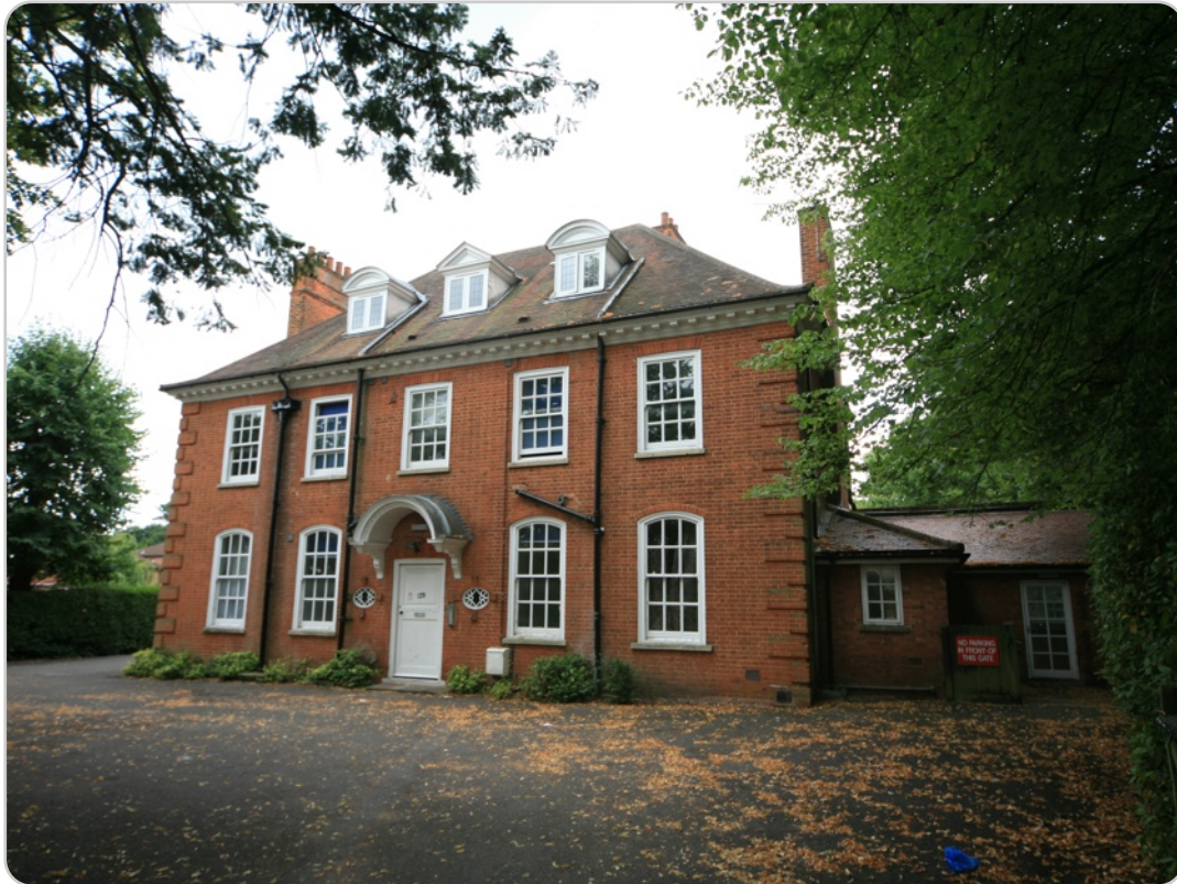
Brighstone House (N elevation) 123 Reading Road, Farnborough
