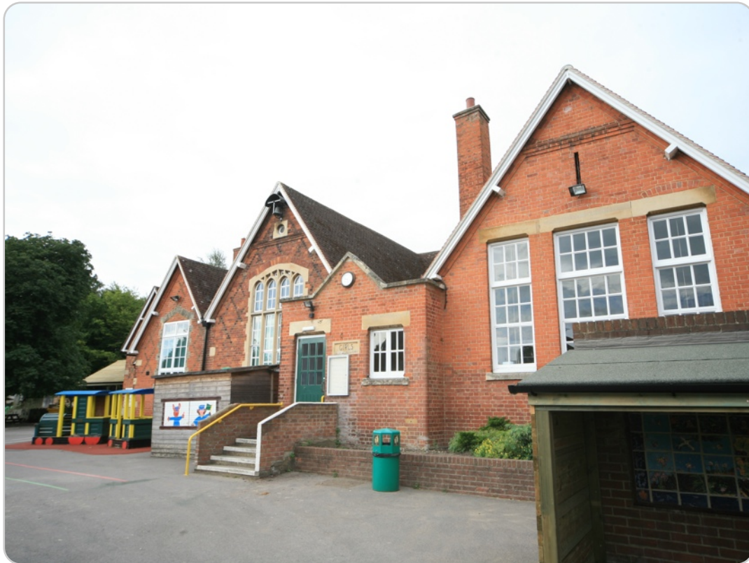
North Farnborough County Infant School (E elevation) Rectory Road, Farnborough
