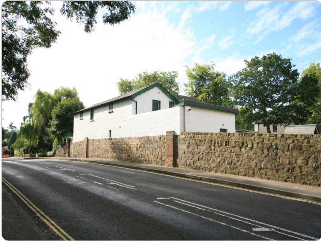
Wall forming part of Fernhill Cottage (N elevation)
