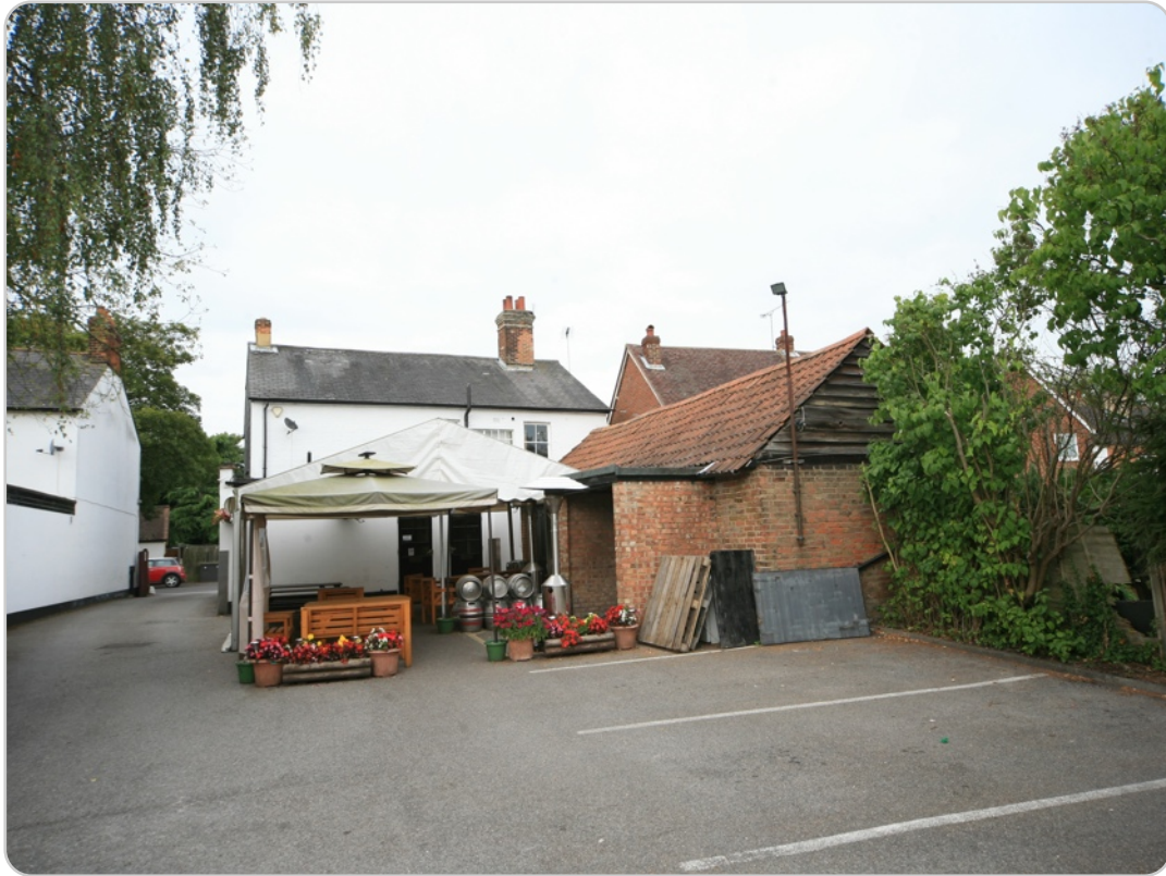
Prince of Wales (E elevation & outbuilding) 184 Rectory Road, Farnborough
