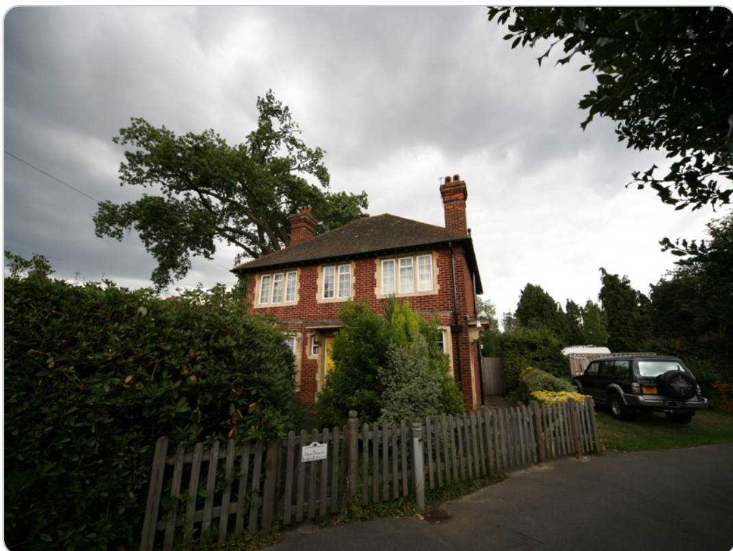
Ship Lane cemetery lodge (W elevation) 154 Ship Lane, Farnborough
