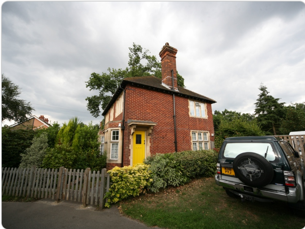
Ship Lane cemetery lodge (S elevation) 154 Ship Lane, Farnborough
