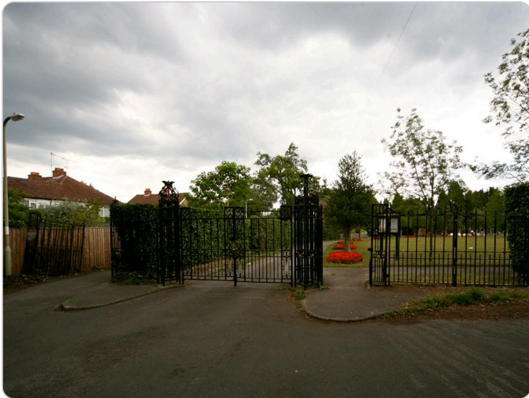
Ship Lane cemetery railings and gates
