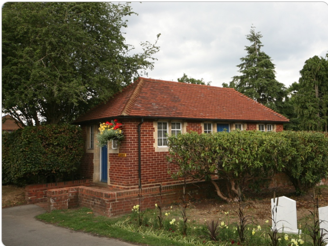
Ship Lane cemetery toilets (SW corner)
