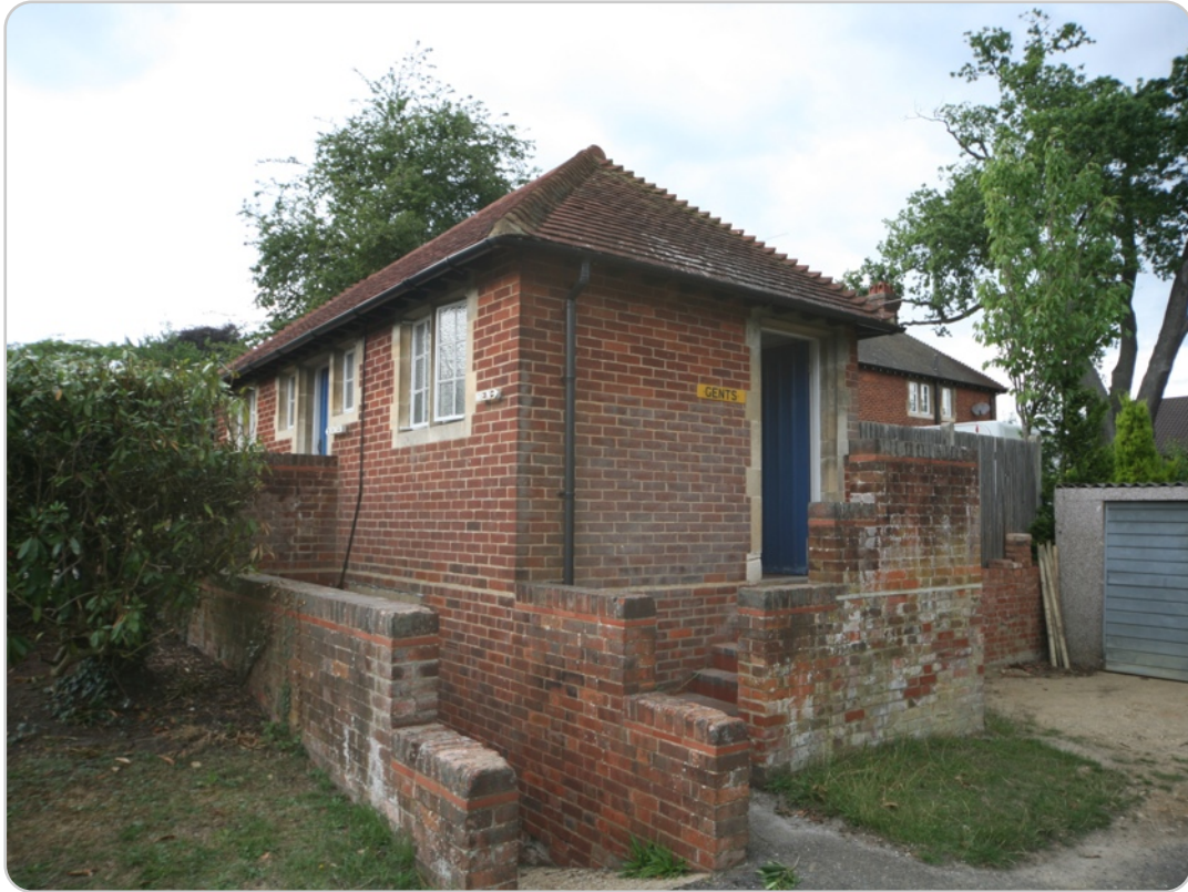
Ship Lane cemetery toilets (SE corner)
