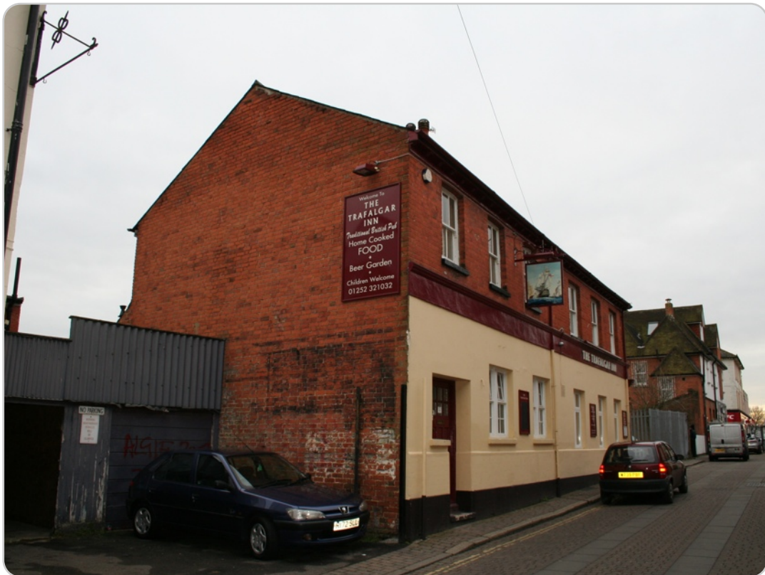
The Trafalgar (NW corner) 1 Short Street, Aldershot
