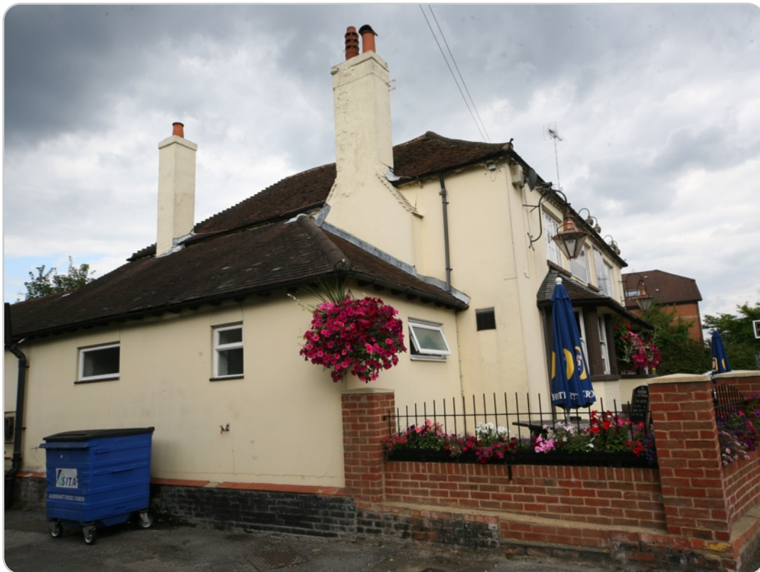
The Old Courthouse (W elevation)
