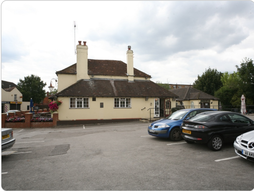
The Old Courthouse (E elevation)
