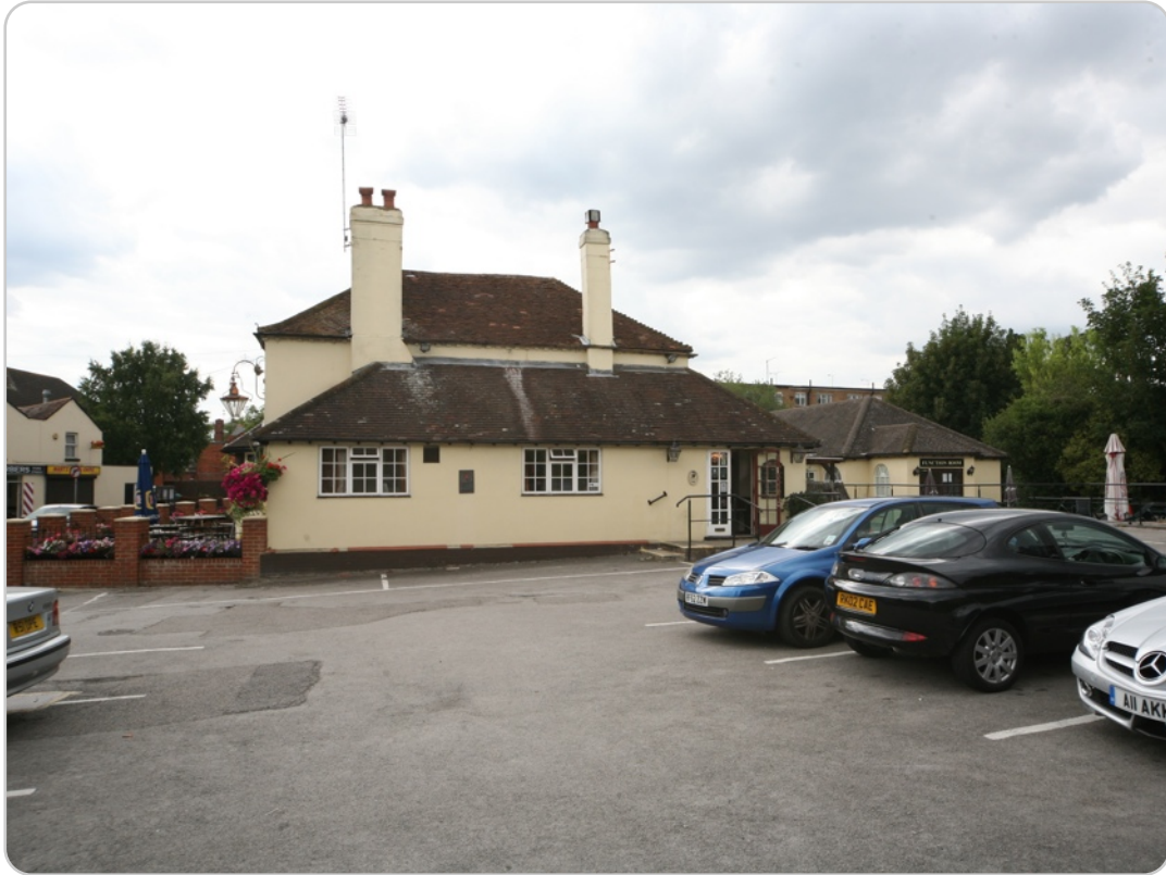
The Old Courthouse (E elevation)
