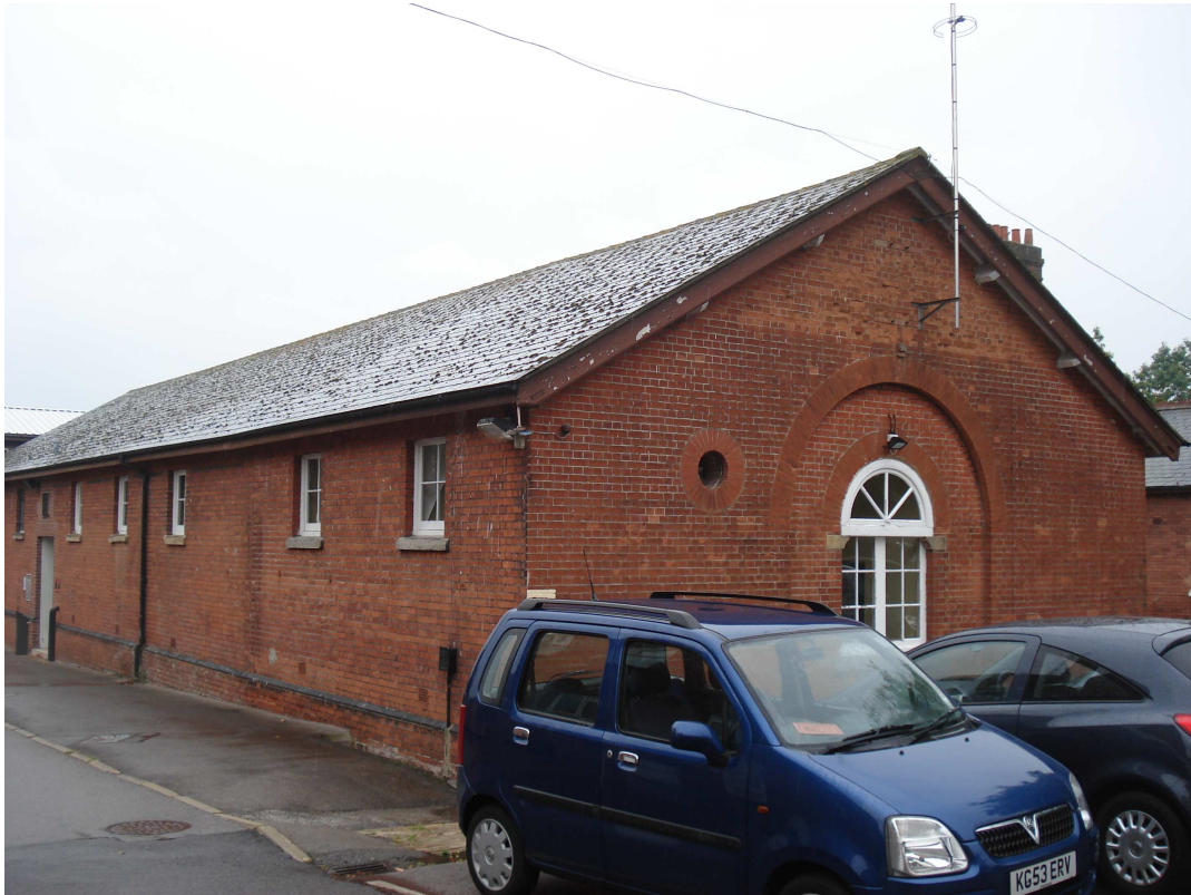
Former stables, Headquarters, Steeles Road, Aldershot – south and part west elevation
