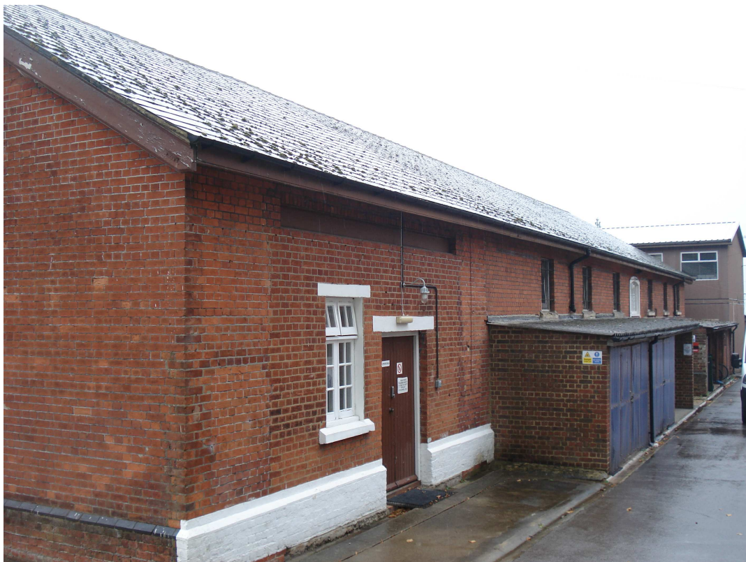
Former stables, Headquarters, Steeles Road, Aldershot – east elevation
